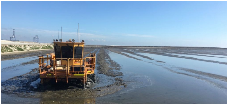
AMC operations in dredged materials
