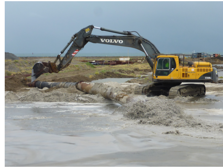
Hydraulic sand placement on AMC managed dredged materials
